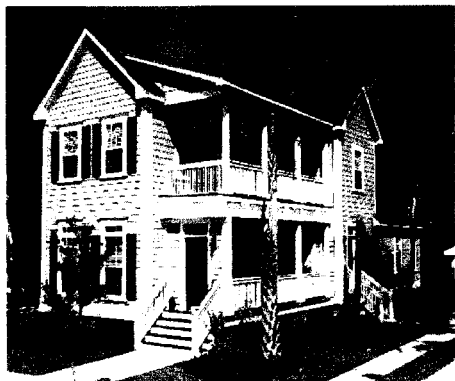
Typical Building Style (Allendale Unit)
