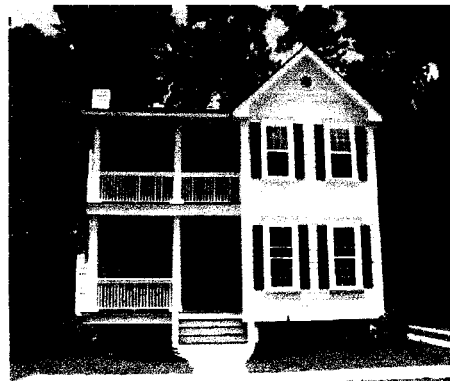
Typical Building Style (Oglethorpe Unit)
